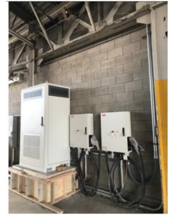
2x 450 kW overhead bus chargers and 3x 50 kW bus depot chargers
