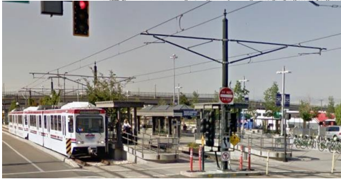
TRAX line, predictable MW-level pulsed load
